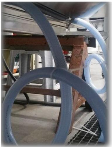
The collection tank, drains and siphons must be kept clear of deposits, mud or dust that could obstruct the normal flow of condensates or other natural seepage.
