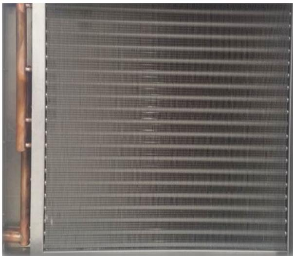
Heat exchangers must always be kept clean to maintain maximum heat exchange. Dust and any other debris should be cleaned off the fins.
