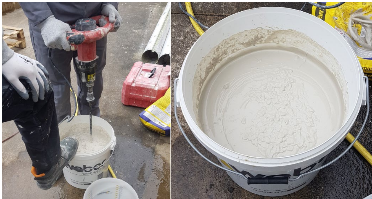
Figure 36: Mixing the sealant
